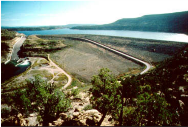
Figure 5. El Vado Reservoir.
